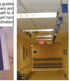
Color coded ceiling guides snap onto T bars and provides a clear path to a heavily trafficked yet hard to find destination
